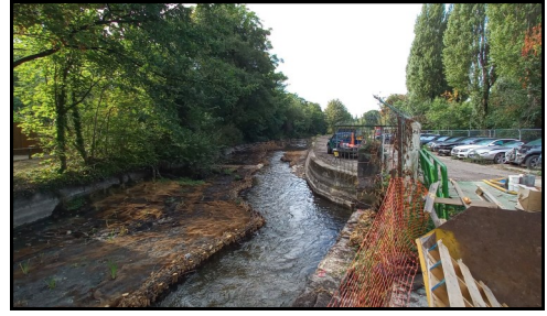
Goat Bridge improvements
